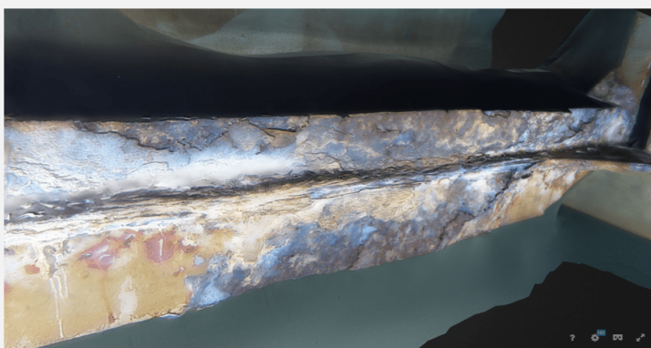
Support Corrosion
