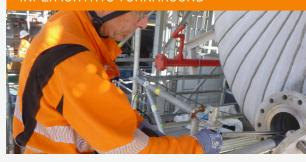
Over two years, Vertech reviewed every item of equipment scheduled for internal inspection of pressure equipment to determine suitability and applicable inspection tooling. They developed an execution strategy for remote visual inspection, provided all RDVI teams for three facilities, and worked with other inspection service personnel to achieve INPEX inspection goals.
