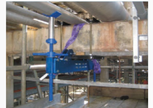
Pipe Rack Jack System
