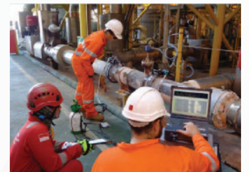
Sonomatic inspectors carrying out Chime Inspection
