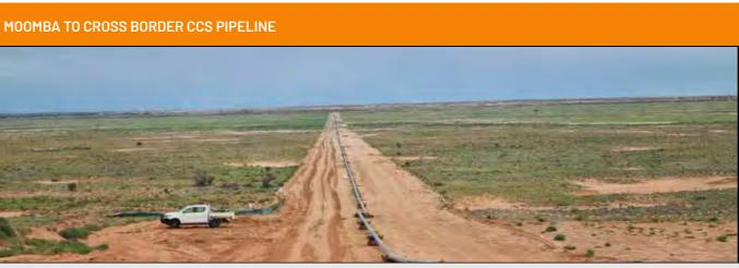
The Moomba to Cross-Border CCS Pipeline runs east from the Santos-owned Moomba gas Plant to depleted reservoirs in the Marabooka and Strzelecki fields. At a diameter of DN250 (10") and a length of approximately 50 kilometres, Vertech was engaged to conduct radiographic inspections throughout the pipeline's construction by MPC Kinetic.
