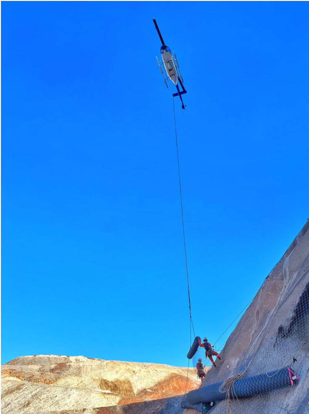
Installing TECCO rolls stage 1 west
